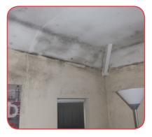
Black spot mould following condensation to walls and ceiling.
